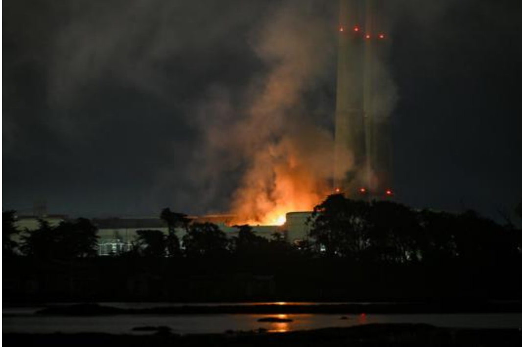
A fire erupted at Moss Landing Power Plant in California on January 17, 2025. Tayfun Coskun/Anadolu via Getty Images© Tayfun Coskun/Anadolu via Getty Images
